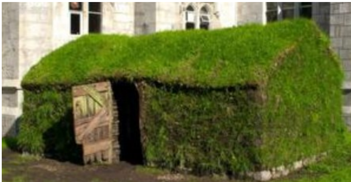
Figure 1: A famine hut made with branches and earth sod
